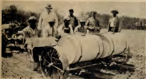
Two-row tractor drawn transplanter used for setting large acreage.
